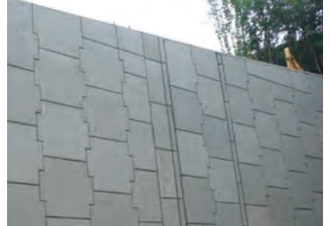
Working on i-Construction
