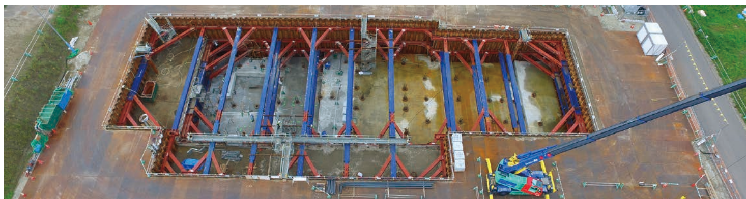
Earth-retaining construction【Hirose twin beam】
