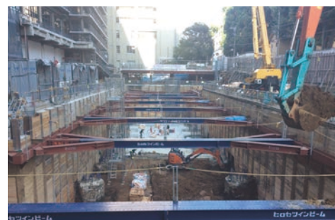
Earth-retaining construction【Hirose twin beam】
